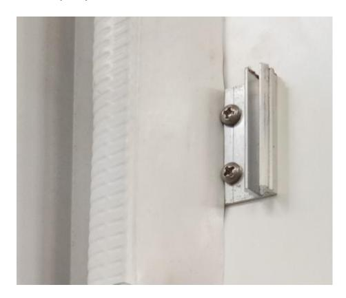
Step 11: Install screen door: Align the fixing block and the mounting slot of screen door, use a rubber hammer to tap the screen door into the mounting slot.
