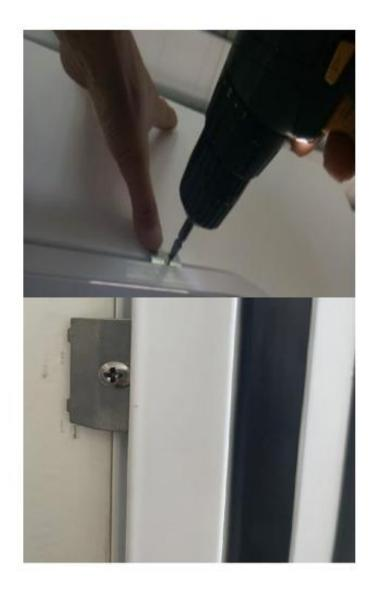
Step 5: Drill holes at the hinge position and screw the hinge with 4x35 stainless steel countersunk head self tapping screws.
