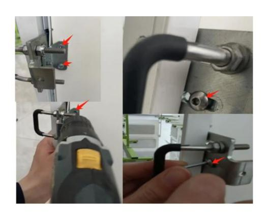
Step 10: Fixing block tightly against the door frame, drill holes on the vehicle body based on the fixing block hole, and screw fixing block with 4x16 self tapping screws.
