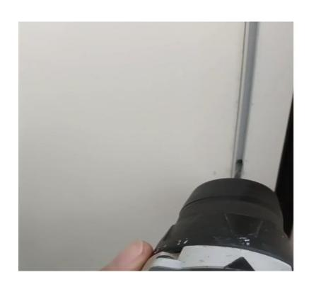
Step 2: Apply sealant evenly along the groove on the inner side of the door frame back.
